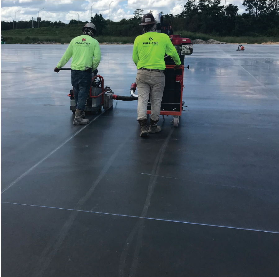
Properly timed saw-cutting of joints in a PLC (Type IL cement) concrete slab
